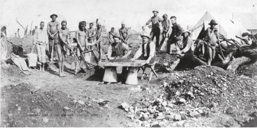
A day in the life of the diggers.
