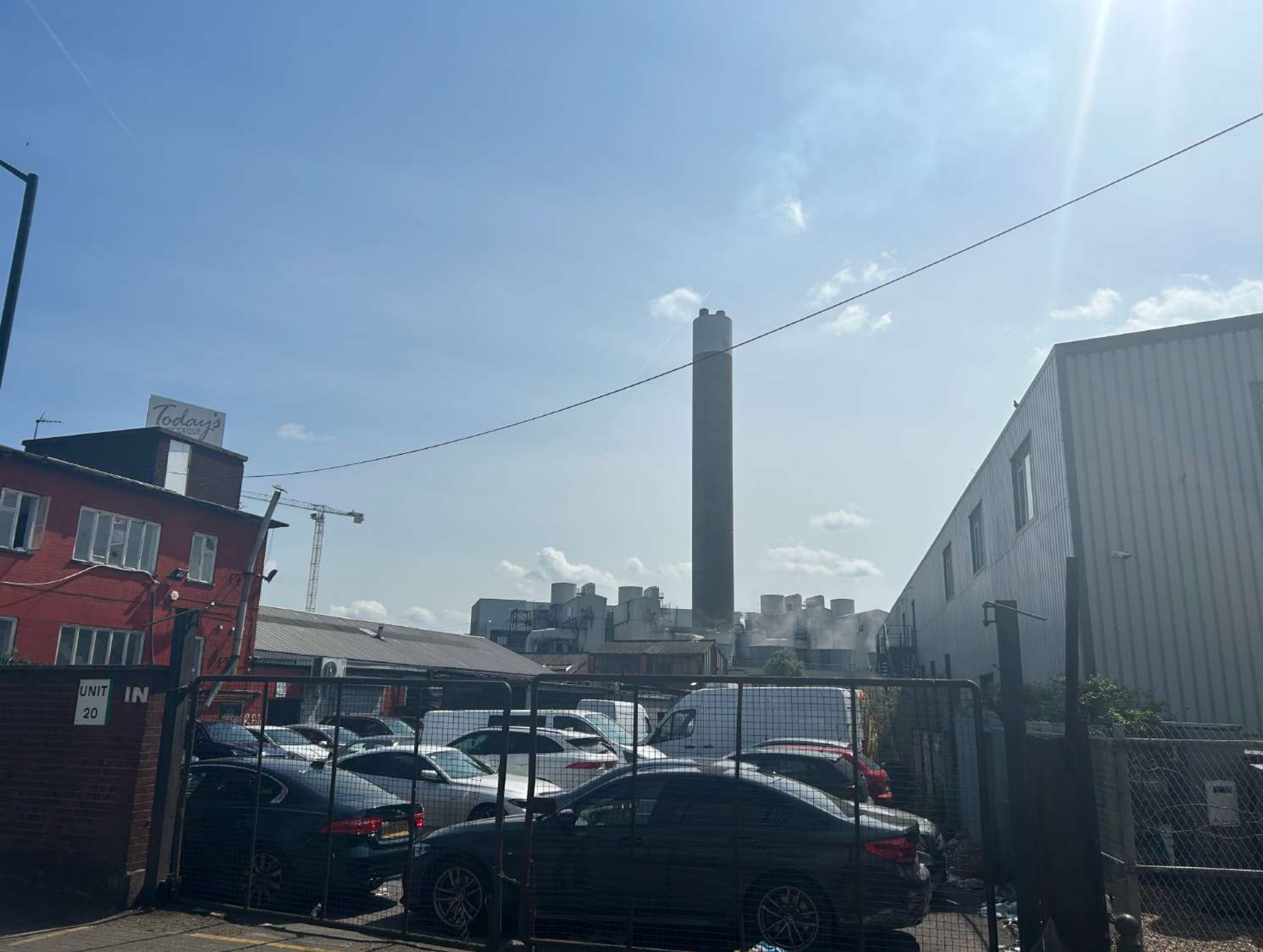
Edmonton Waste Incinerator, 2024
